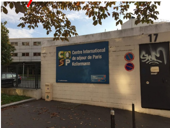
← CIS Kellermann is a big white building with the name on it
